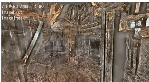
Figure 1.8 – Possible corium relocation into the primary containment vessel in Fukushima Dai-ichi unit 2
